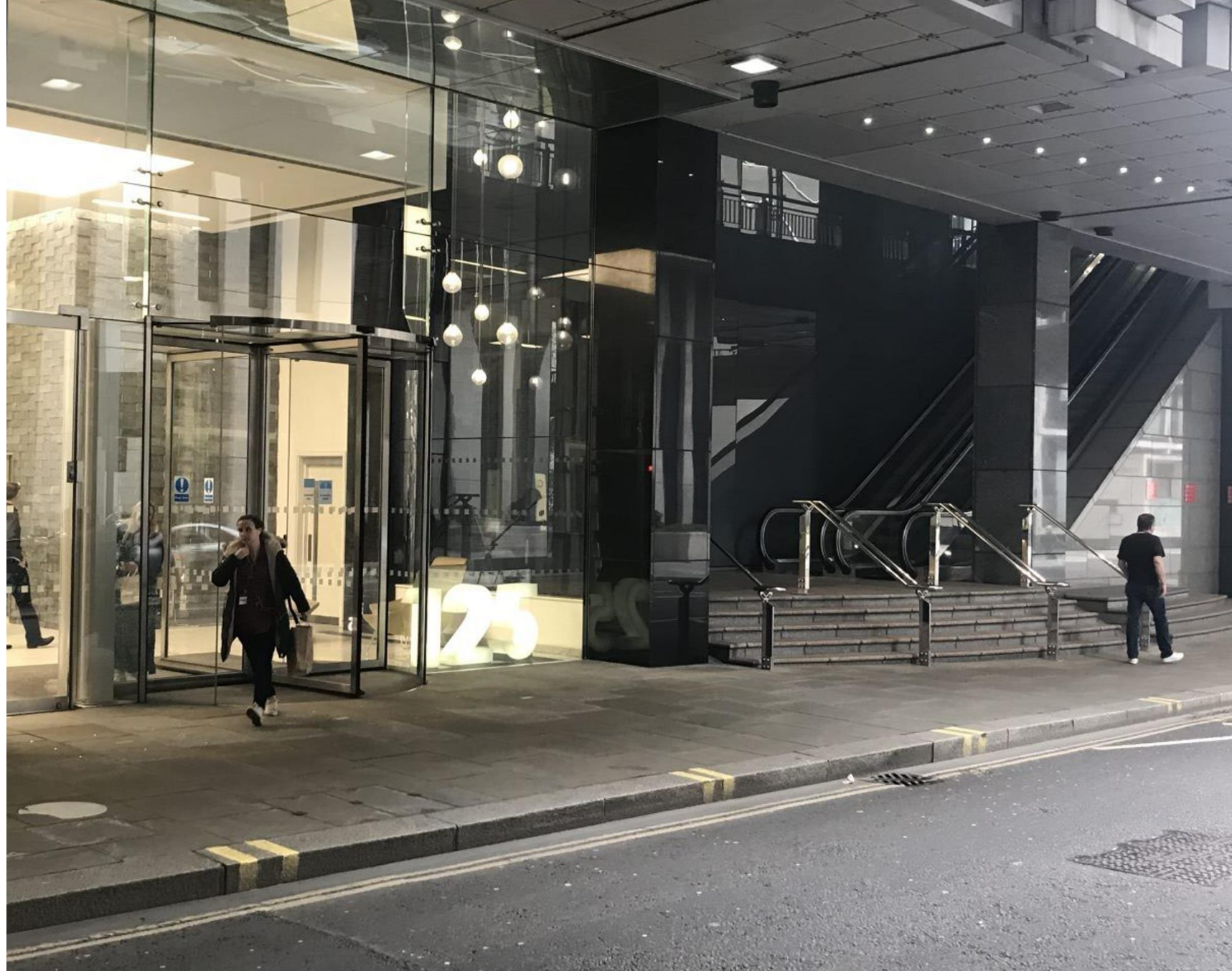
Existing Site Photos Wood Street (north side)
