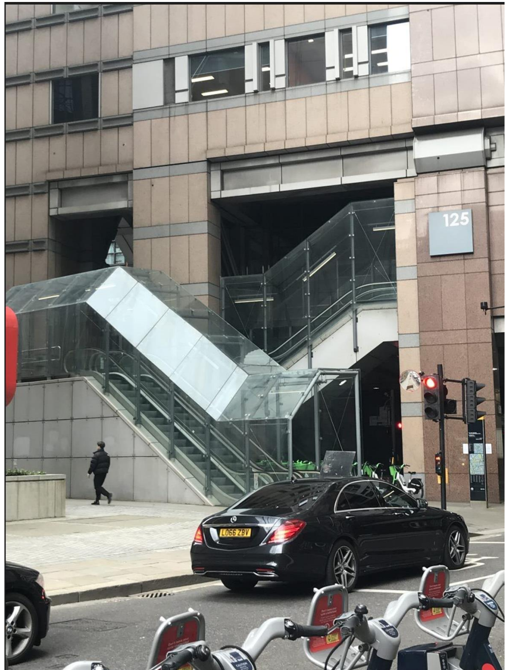
Existing Site Photos Wood Street (south side)
